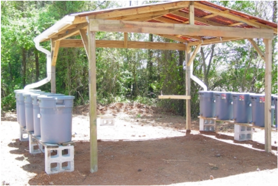
Figure 15. A water catchment can provide enough water to soak 90 logs with just one inch of rain. The surface area of this catchment is about 143 square feet and it will collect 89 gallons of water from one-inch of rain.
